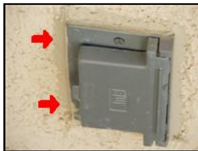
3.4 Picture 1 Breach Sealed
