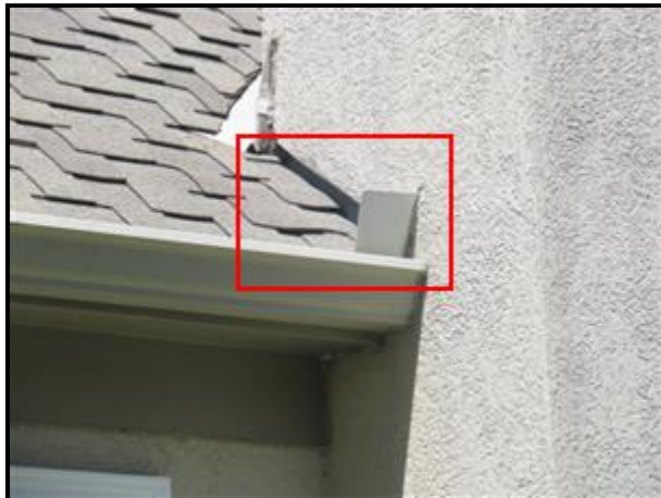
4.5 Picture 3 New Add-On Kickout
