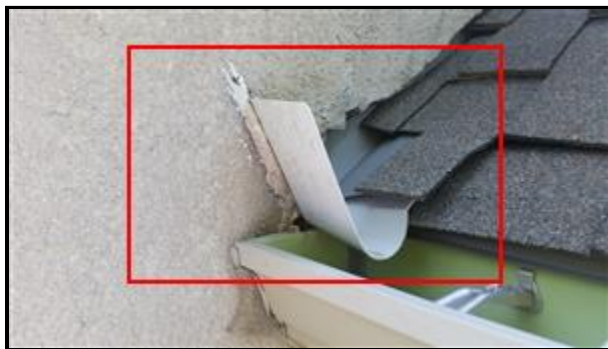
4.5 Picture 7 New Poor Kickout
