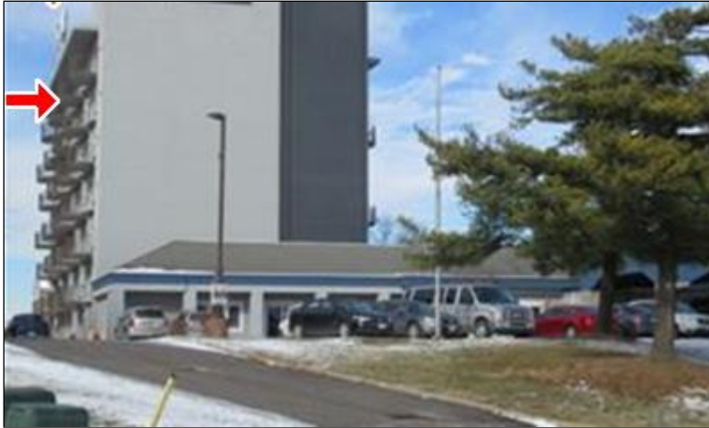
11.0 Picture 1 Tower (not inspected)
