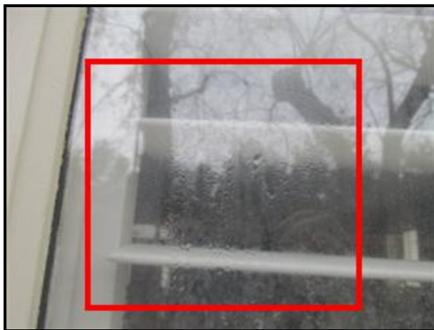
5.1 Picture 1 Deck Door
