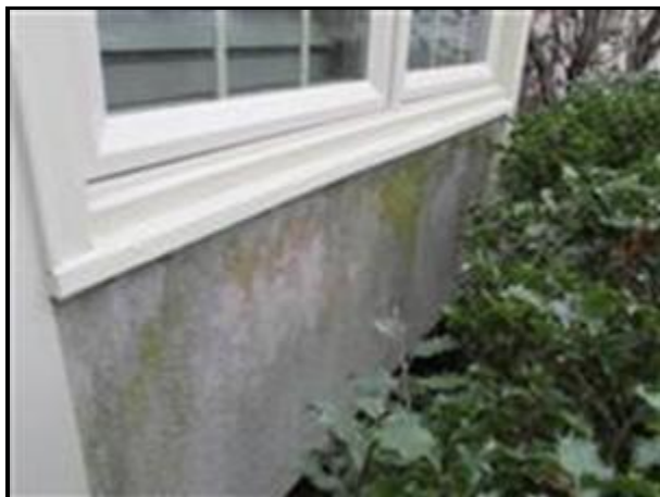
9.1 Picture 1 Front Wall - Right of Entry
