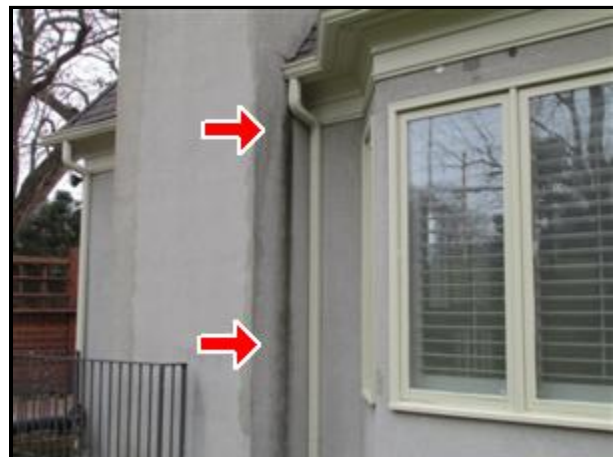
9.1 Picture 2 Chimney on Left Side
