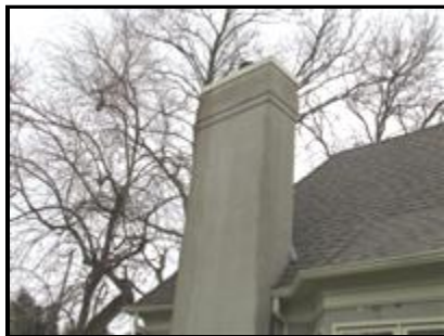
4.0 Picture 1 Left Chimney
