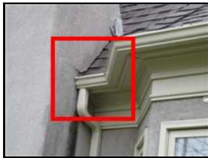
4.5 Picture 2 Left Chimney
