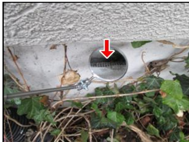
2.4 Picture 2 Plastic Mesh Under Wall
