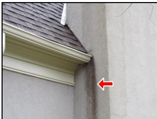
9.1 Picture 3 Chimney / Left Side
