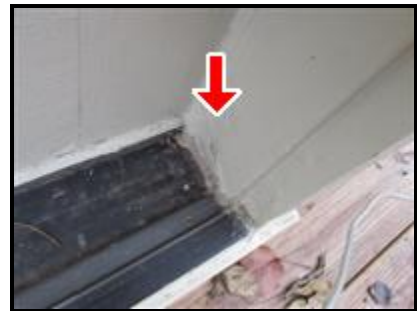
7.0 Picture 3 Deck Door
