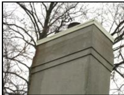
4.0 Picture 2 Left Chimney
