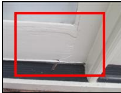
7.0 Picture 2 Deck Door
